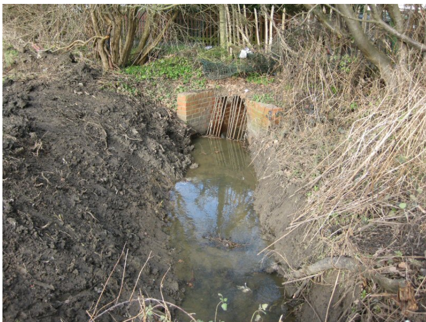
Potters Bar Brook culvert under Ashwood Road
